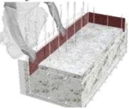
\*In the case of rounded parts and corner constructions, simply bend the AQUAFIN®-CJ7 into the corresponding shape (refer to the image below).
